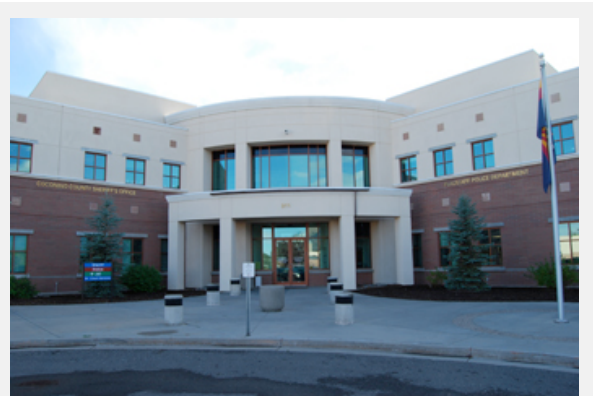
Joint police-sheriff building, Flagstaff, Arizona.
